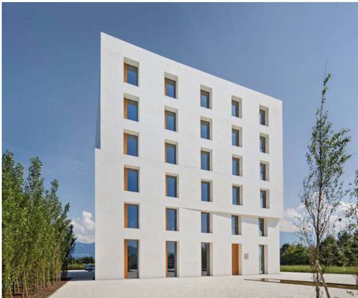
Arch. Baumschlager Eberle – Office building Lustenau (A)
